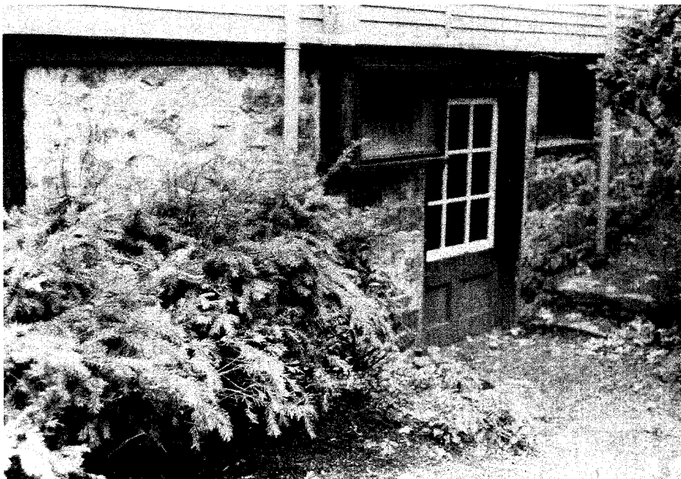
Basement door opening onto the garden.
