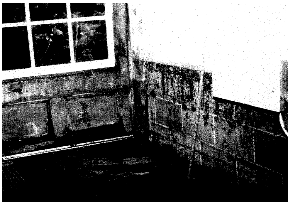
Basement door interior. View inside the mechanical room housing the heating, ventilating, and air-conditioning equipment, showing the flood level in the room which is adjacent to the lower vault and the basement storage room.
