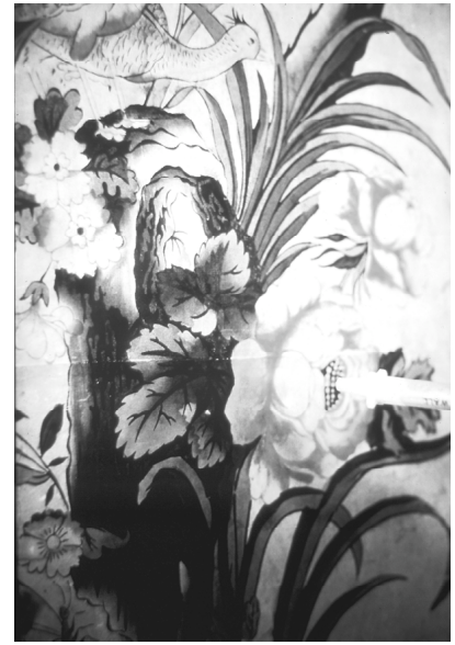
Fig. 6. Blackwell vestibule, during treatment: wetting water stain with ultrasonic mist
