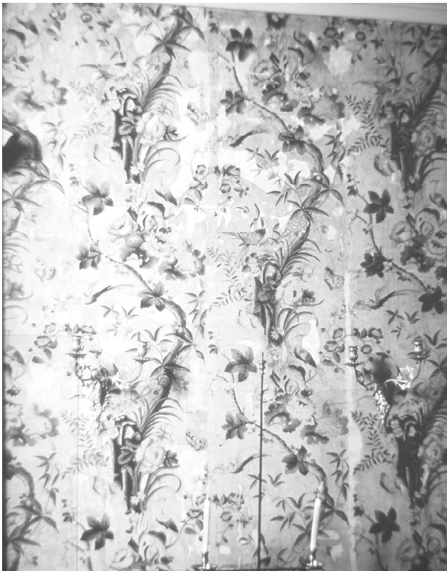
Fig. 9. Blackwell vestibule south wall, before treatment
