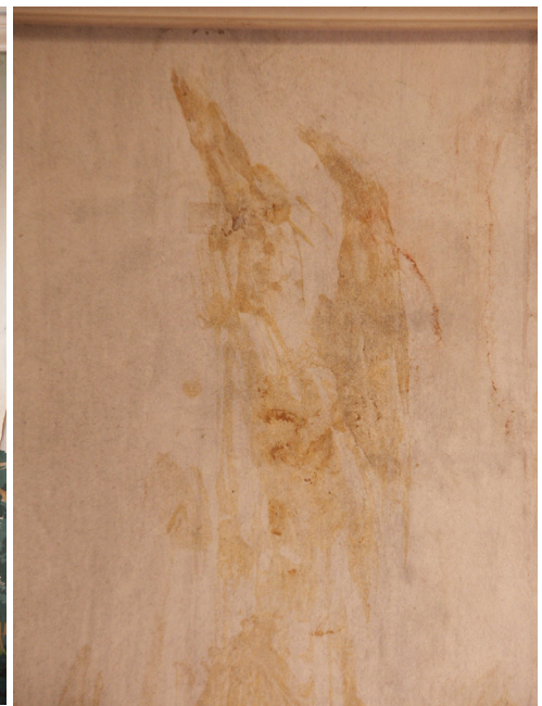
Fig. 5. Rubber cement residue left on the plaster after the removal of the wallpaper panel visible in figure 4
