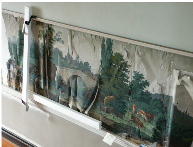
Fig. 3. The torn, partially delaminated wallpaper supported by Styrofoam braces.
