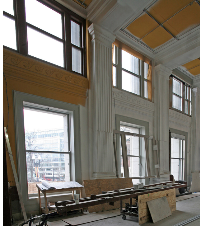
Fig. 8. South facing historic windows.
