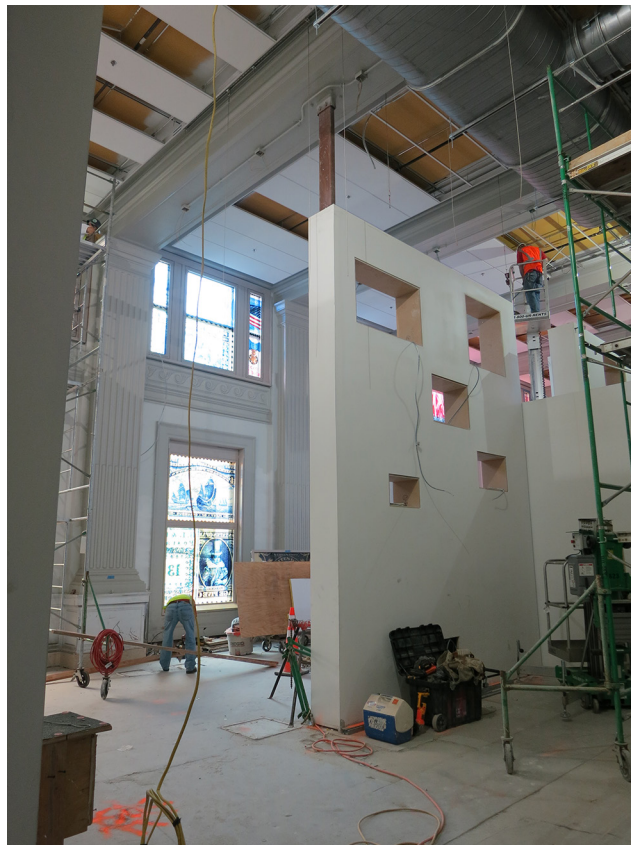
Fig. 7. Constructing barrier walls to block sunlight.
