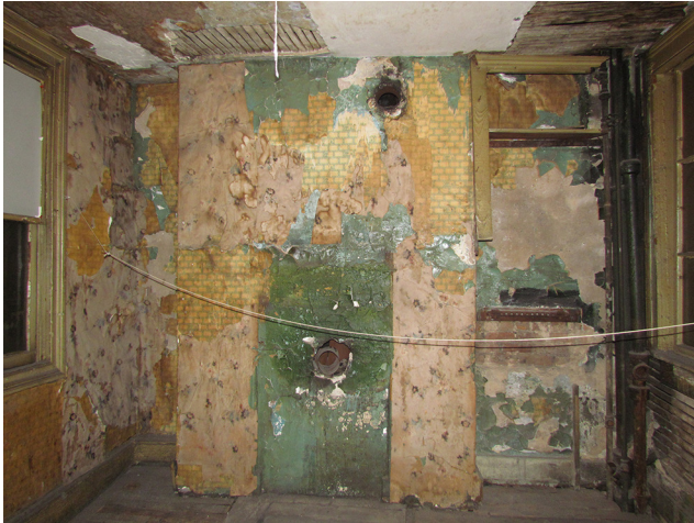
Fig. 5. “Preserved” kitchen of Apartment 11.
