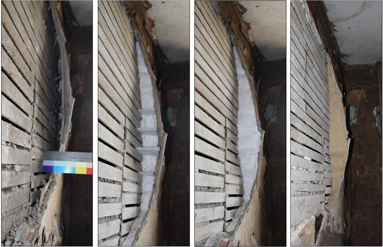
Fig. 7. Stabilization of the plaster substrate to prevent additional wallpaper loss.
