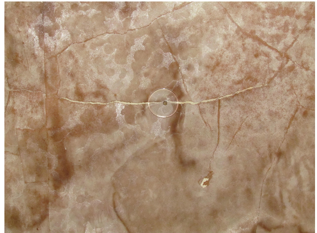
Fig. 6. A pin placed along a tear to prevent puncturing the wallpaper.
