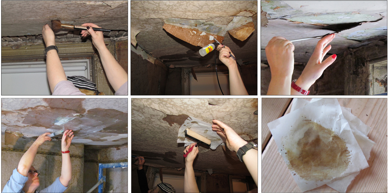
Fig. 8. Process of wallpaper stabilization using Tri-funori includes cleaning, consolidating, re-adhering, saturating, flattening, and cleaning.
