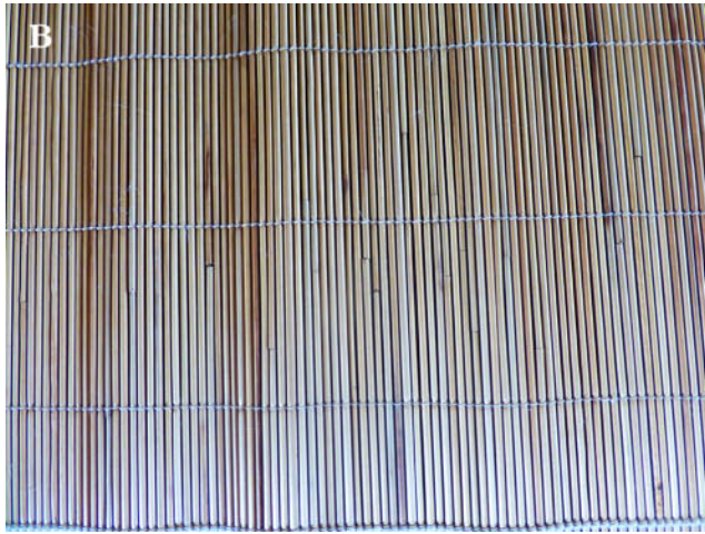
Fig. 23b. Detail of a kaya screen showing the random placement of laid support joints.
