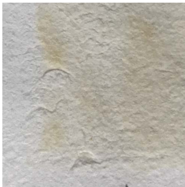
Fig. 12. Fiber damage from overwetting.
