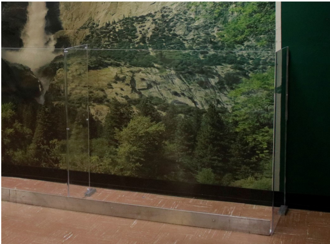
Fig. 13. Barrier showing bent Plexiglas sheets, feet, and kick plate.
