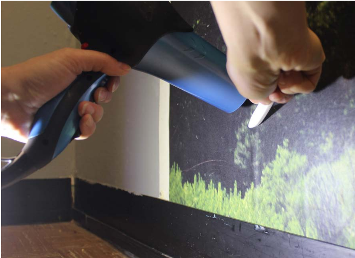
Fig. 10. Using heat from a hair dryer and Teflon folder to remove minor bubbling.
