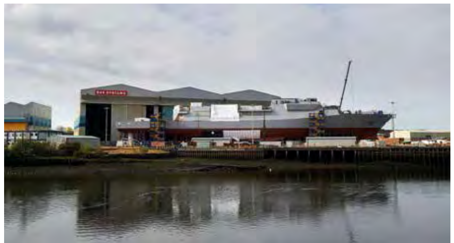
The constituent blocks of HMS GLASGOW were joined together at the start of May 2021.
