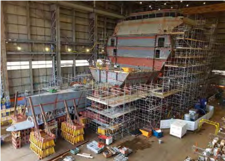
Type 26 production has been allocated to BAE Systems' shipyards on the River Clyde, where this image of the forward block of lead ship HMS GLASGOW was taken.
