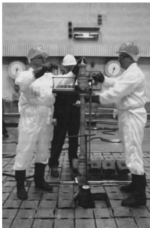
Figure 2: Loading fuel elements into a channel while the reactor was operating. Source: Radiant Power Engineering. Siberian AES: History with Continuation , 2008.
