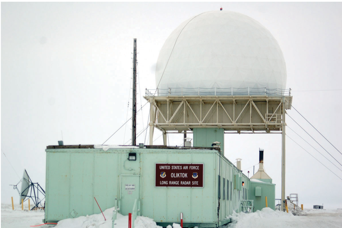
Figure 10: Oliktok Long Range Radar Site
