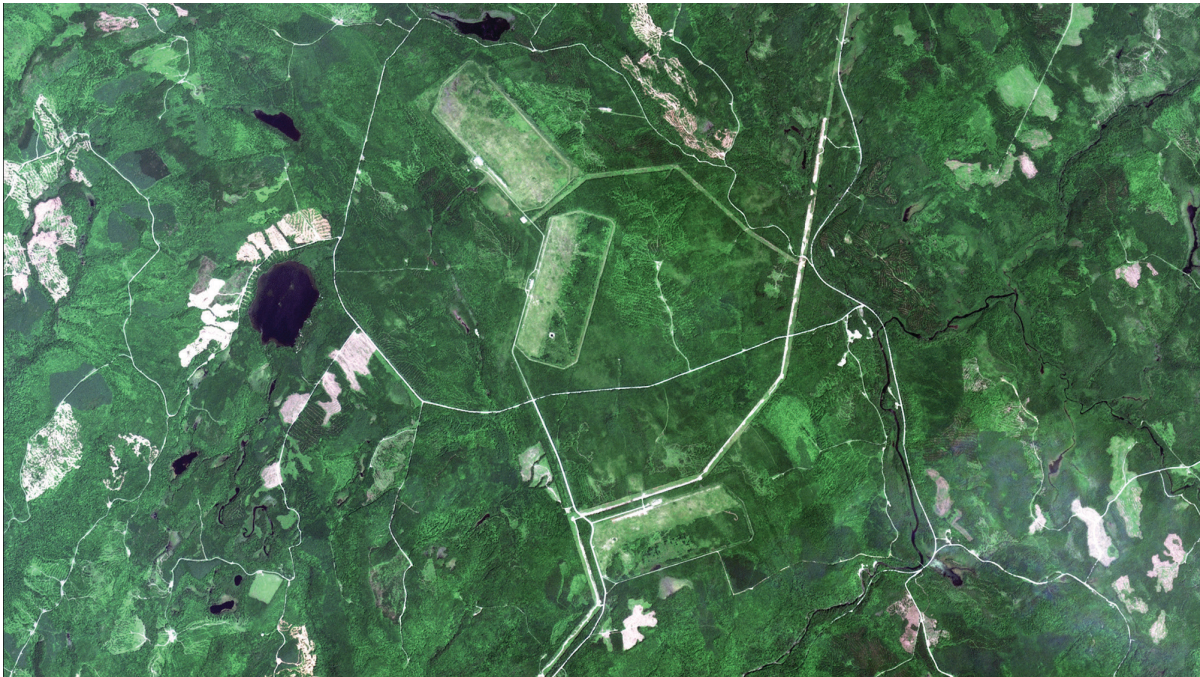
Figure 36: Abandoned Cold War OTH-B Arrays near Moscow, Maine
