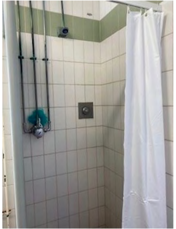
Showers in dormitory block
