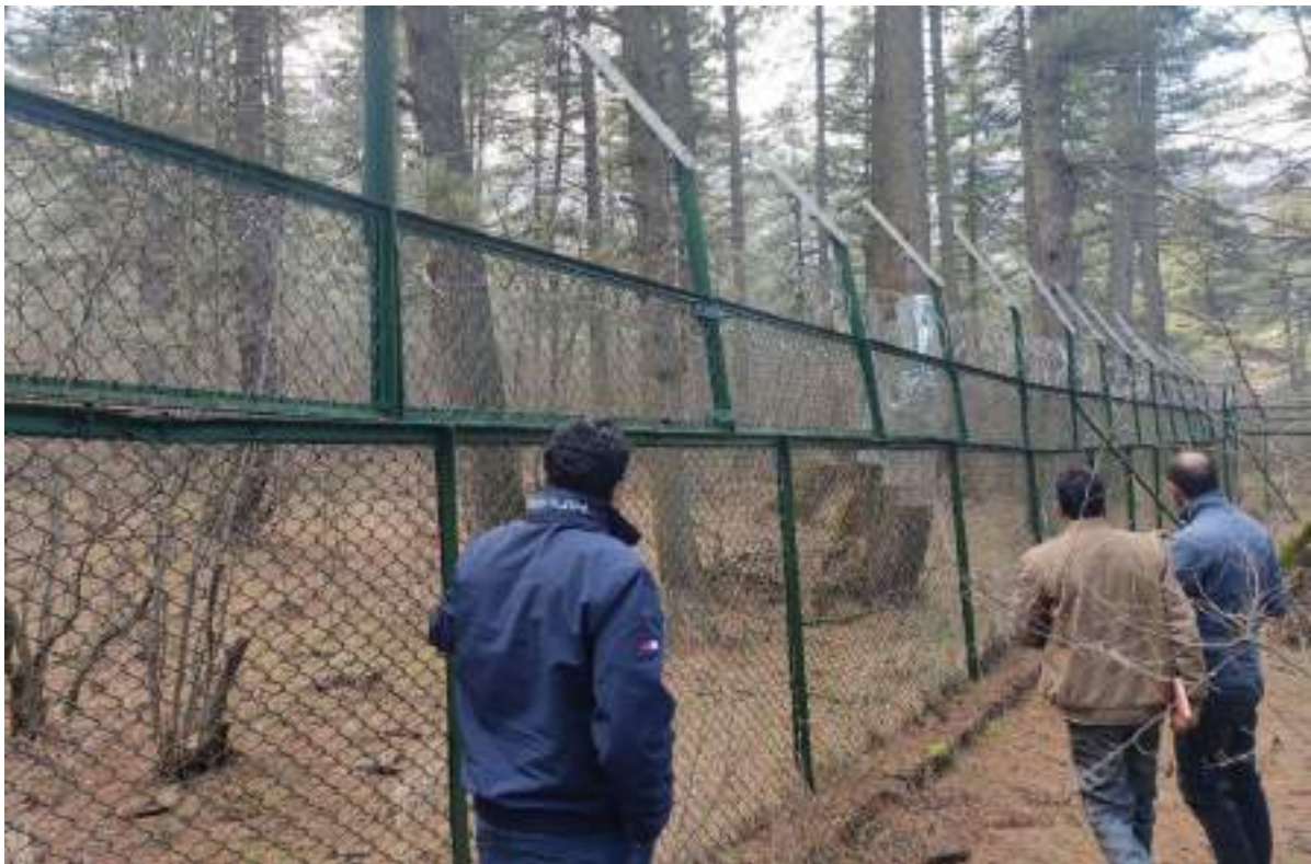
Fig 3: Fence at the Enclosure II
