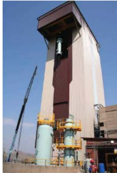
The Helium Test Facility (HTF)
