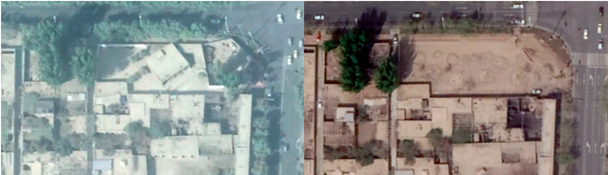
Figure 7: A mosque in Hotan's Karakash County, before and after 2017
