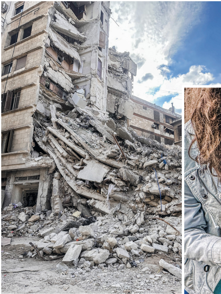
[LEFT] Earthquake destruction in Aleppo, Syria in February 2023
