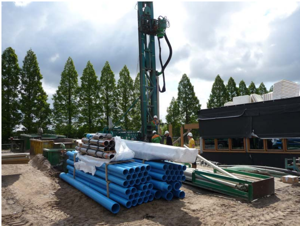
Figure 3 Drilling process NIOO
