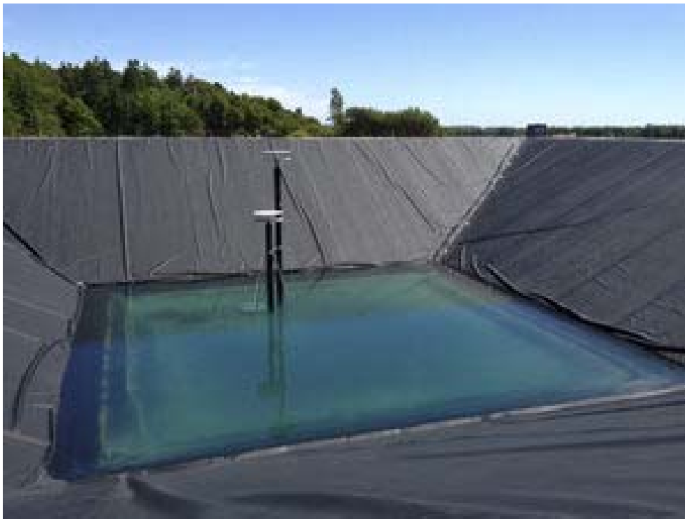
Figure 4.1 Picture of Dronninglund Pit Storage under construction. Dronninglund District heating; 37,573 m 2 of solar collectors and a 62,000 m 3 water in pit heat storage (PlanEnergi)
