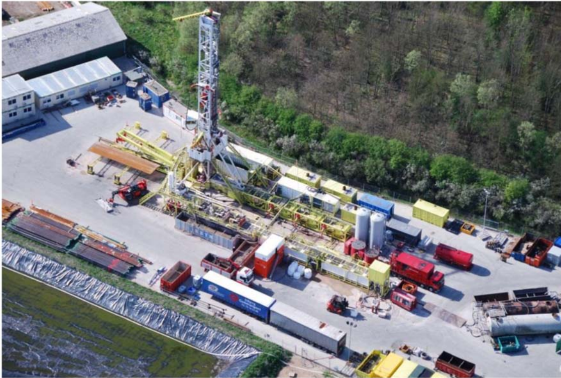
Figure 2.7 Deep geothermal drilling in Sønderborg, Denmark, in 2010 (from 29 )
