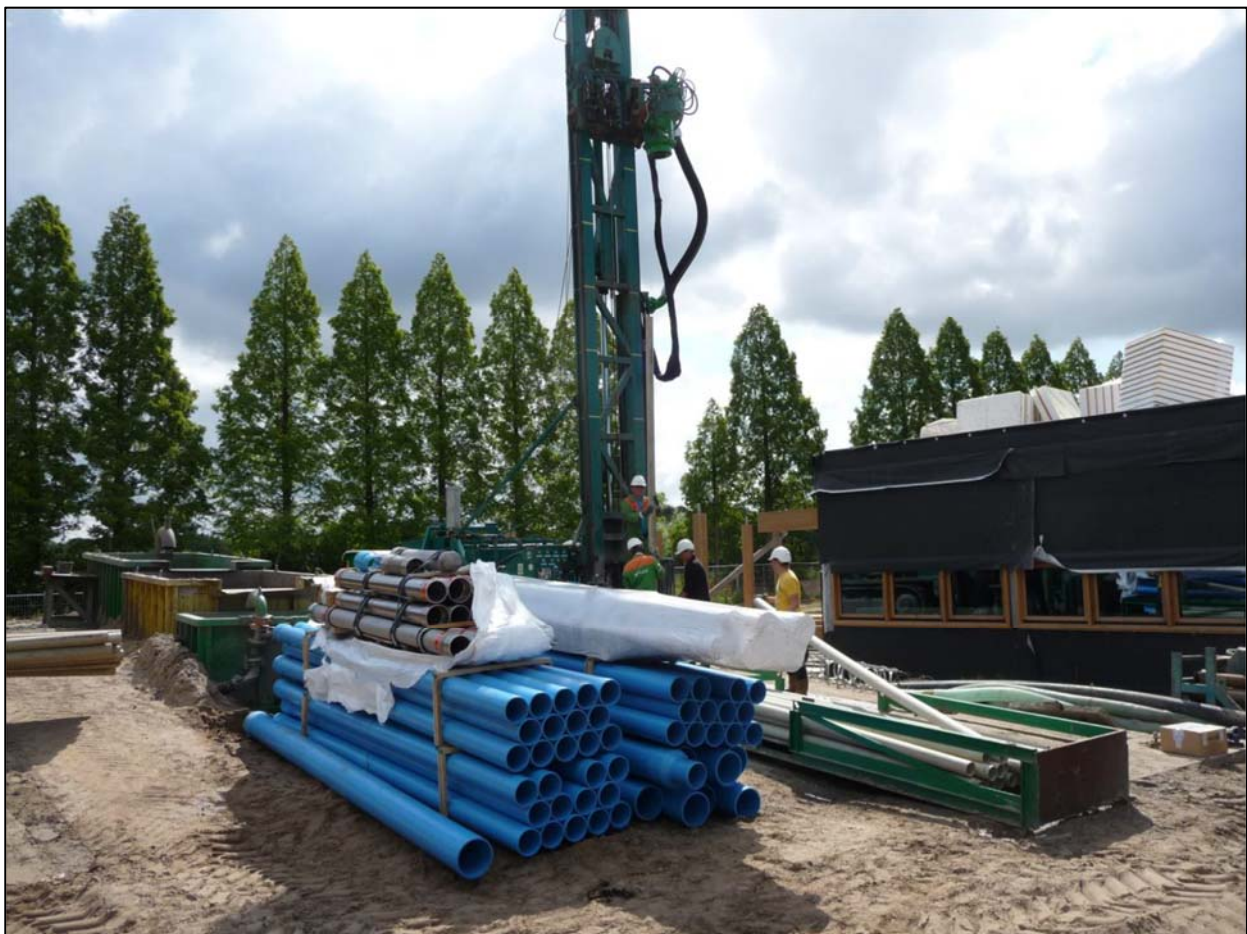
Figure 2.5 Picture from drilling site at the NIOO HEATSTORE case study in the Netherlands (IF Technology)
