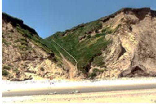
Plate 10 - Eroding soft coast - Co. Wexford
