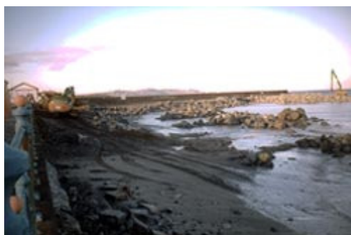
Plate 35 - Coastal protection works
