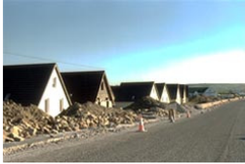
Plate 22 - Holiday home construction - Co. Clare
