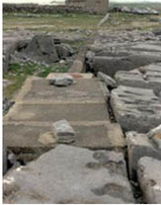
Plate 32 - Sewage outfall at Doolin, Co. Clare discharges onto the foreshore.
