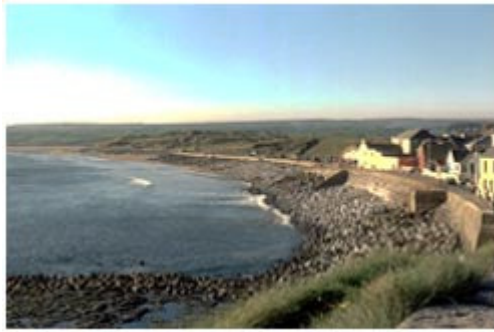
Plate 23 - Coastal protection - Lehinch, Co. Clare
