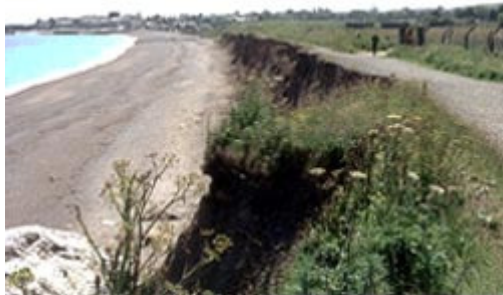
Plate 8 - Coastal erosion north of Greystones - Co. Wicklow
