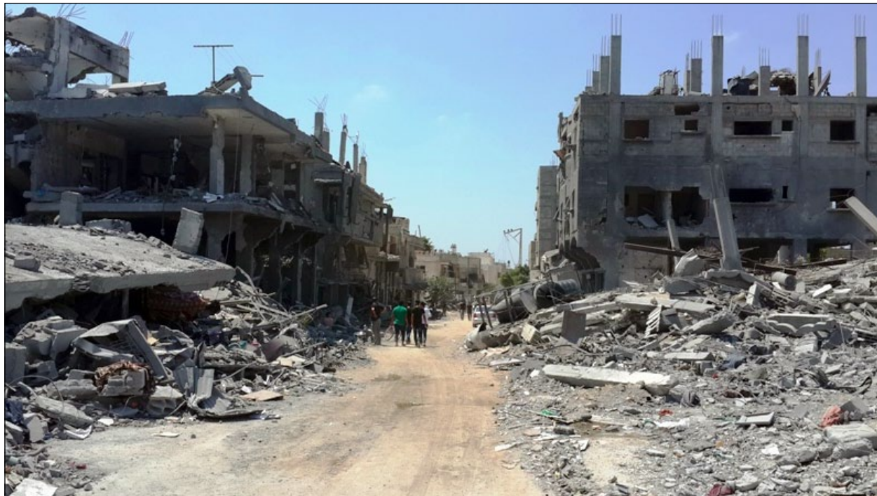
Source: Al-Haq, Houses Demolished in Beit Hanoun during Operation Protective Edge
