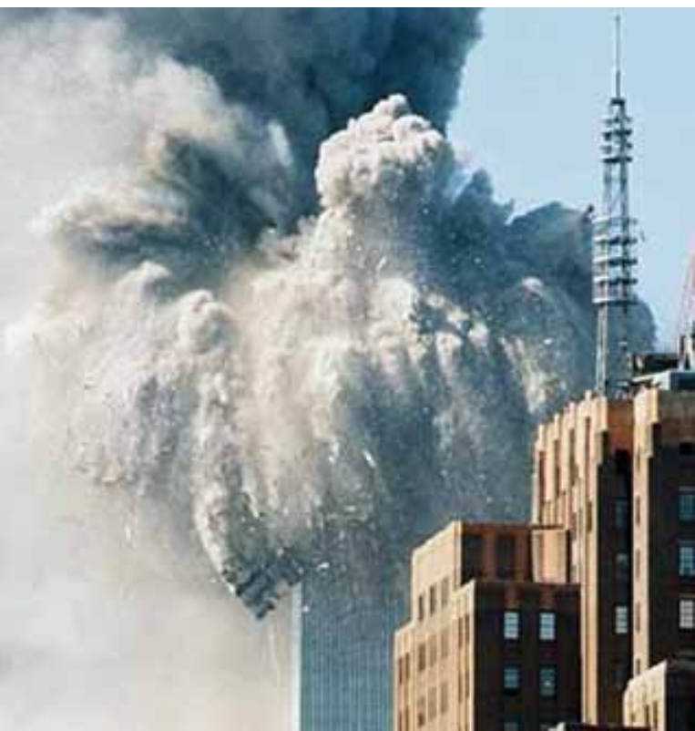
This is the WTC 'collapse'
