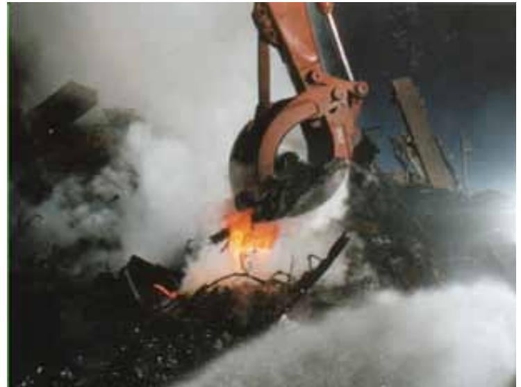
A digger pulls up molten metal debris.
