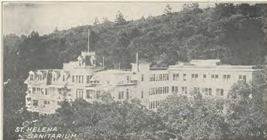
THE MAIN BUILDING—SHOWING THREE OF THE FIVE STORIES New Concrete Hydrotherapy Building at the Right
