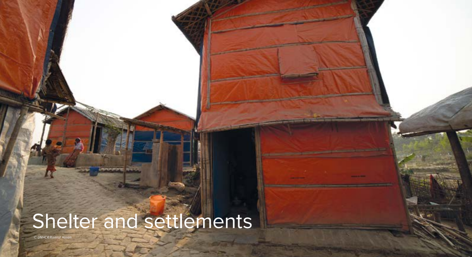
UNHCR is piloting steel-framed double-storey shelters to make better use of space in refugee camps in Cox's Bazar, Bangladesh. The frames can be dismantled and the steel reused when they are no longer needed.
