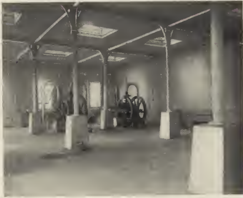
FIG. 37.—INTERIOR VIEW OF THE ENGINE ROOM.
