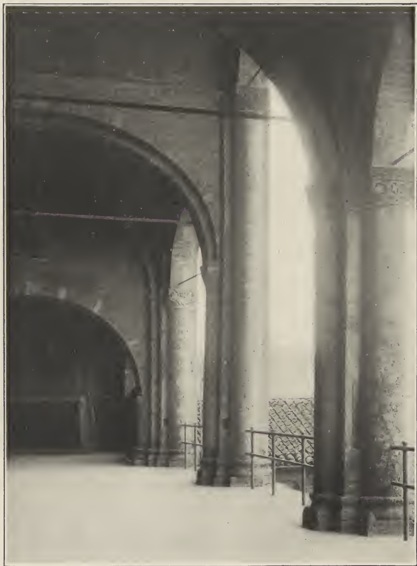
FIG. 9. RETURN CURVE OF THE LEANING FAÇADE OF S. AMBROGIO, MILAN. Taken inside the portico of the second story. Photograph of the Brooklyn Institute Survey, 1901.
