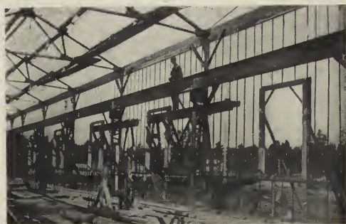
FIG. 28.—FRAMING FOR FACTORY SIDE WALLS.
