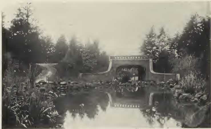
FIG. 4.—BRIDGE, GOLDEN GATE PARK. Built of reinforced concrete.
