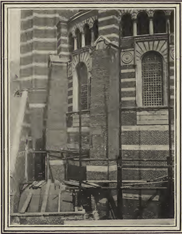
DETAIL OF THE APSE, SHOWING THE VERY GRADUAL OFFSETS OF THE BUTTRESSES.
