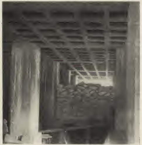
FIG. 32.—UNDERSIDE OF THE COMPLETED FLOOR SUPPORTING THE BINS. Shown in Fig. 30.
