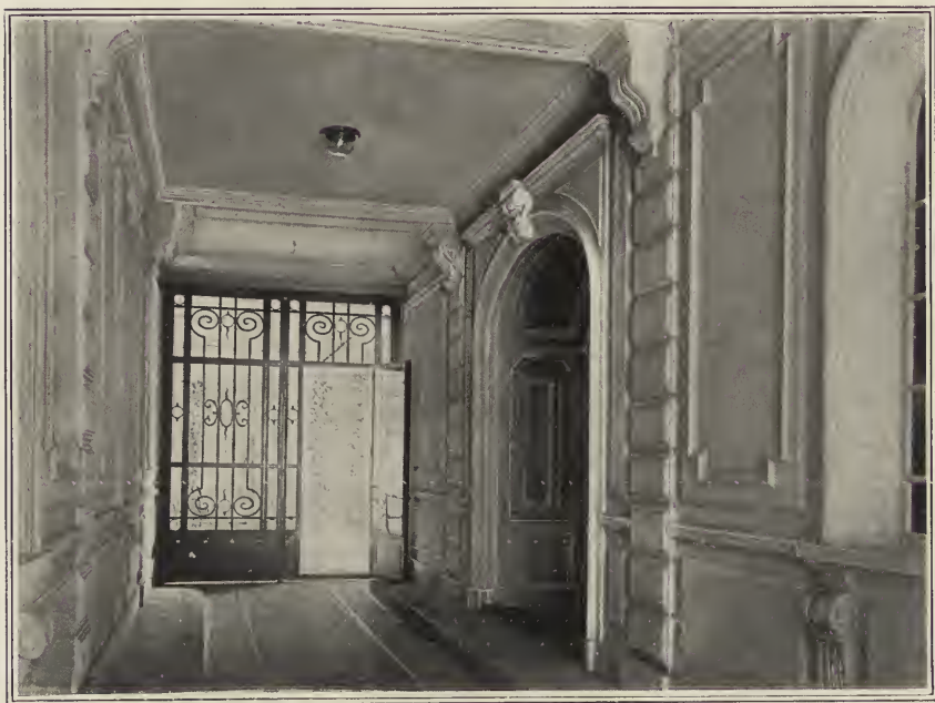
FIG. 13. VESTIBULE ENTERED FROM THE COURT OF THE PRIVATE DWELLING ON THE RUE DE LÜBECK, PARIS.
