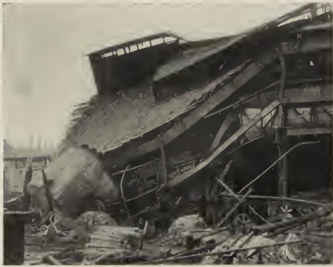
FIG. 18.—THE BEHAVIOR OF UNPROTECTED STEEL IN FIRE.
