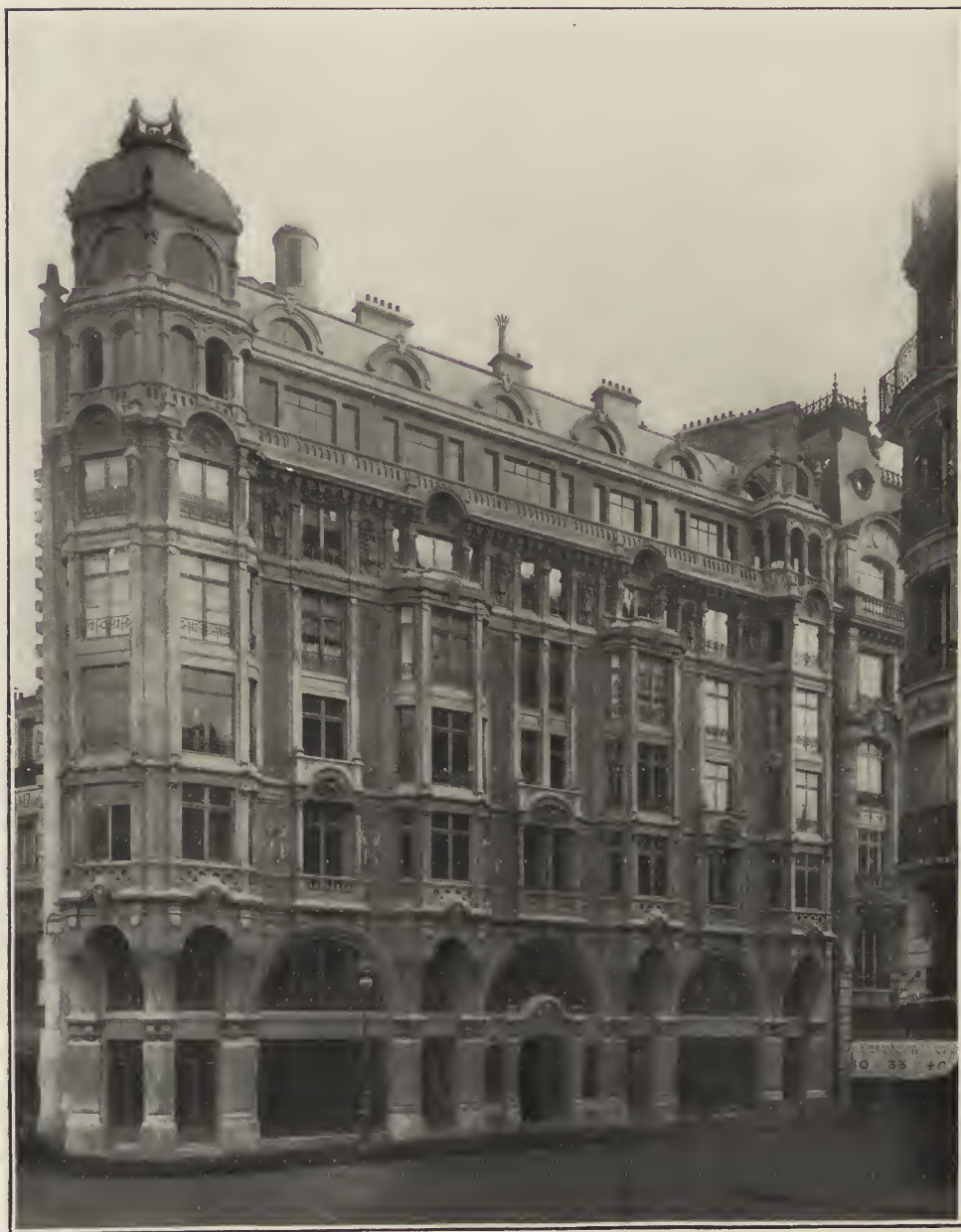
FIG. 2. AN APARTMENT HOUSE AT NO. 1 RUE DANTON, PARIS, DESIGNED BY M. ARNAND AND CONSTRUCTED THROUGHOUT OF CIMENT ARMÉE.
