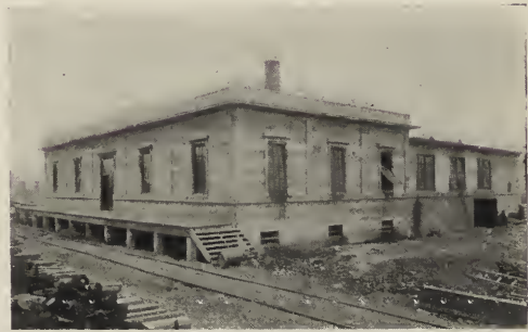
FIG. 36.—THE POWER HOUSE.
