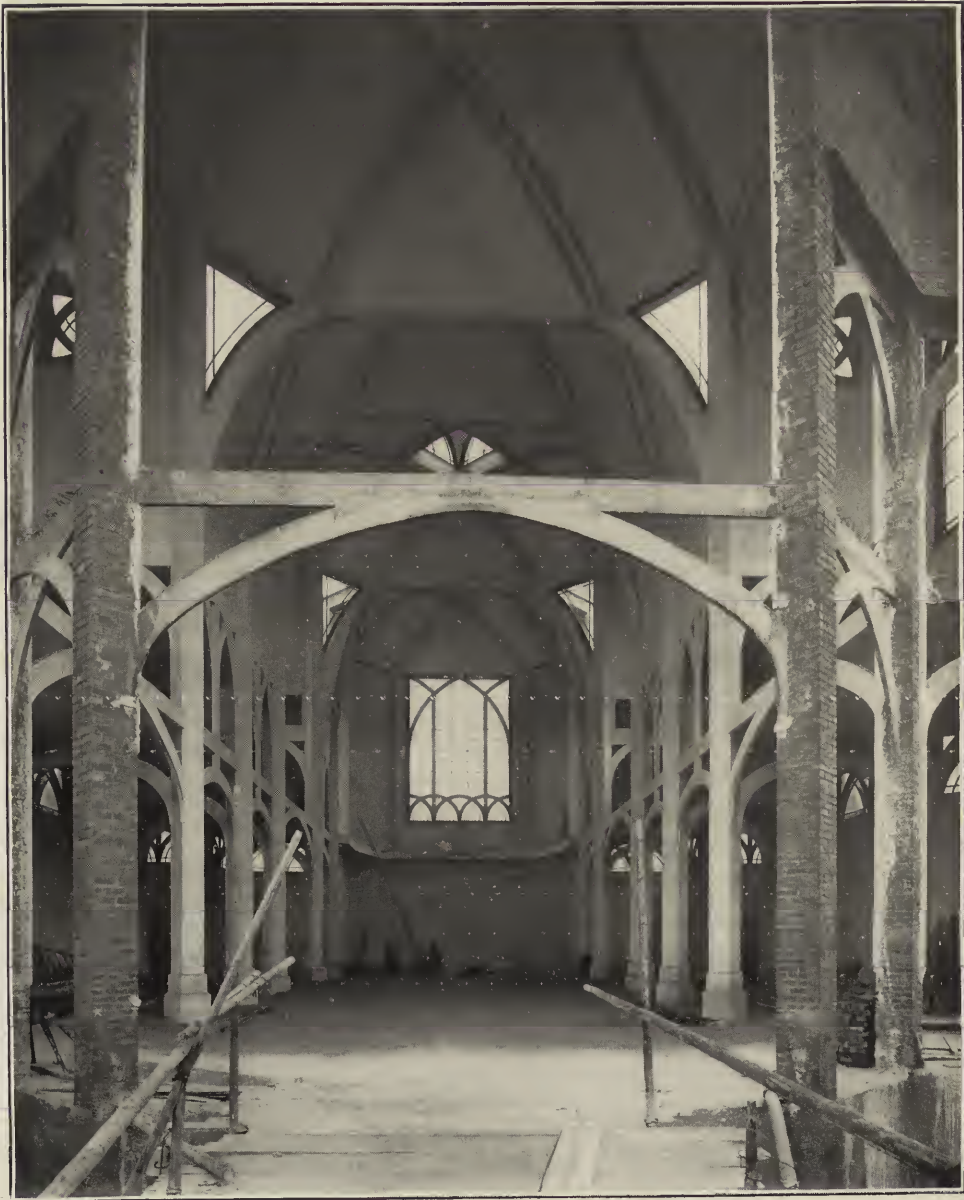
FIG. 7.—INTERIOR OF THE UPPER CHURCH.
