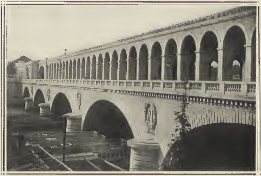
A DOUBLE DECKED BRIDGE IN PARIS.
