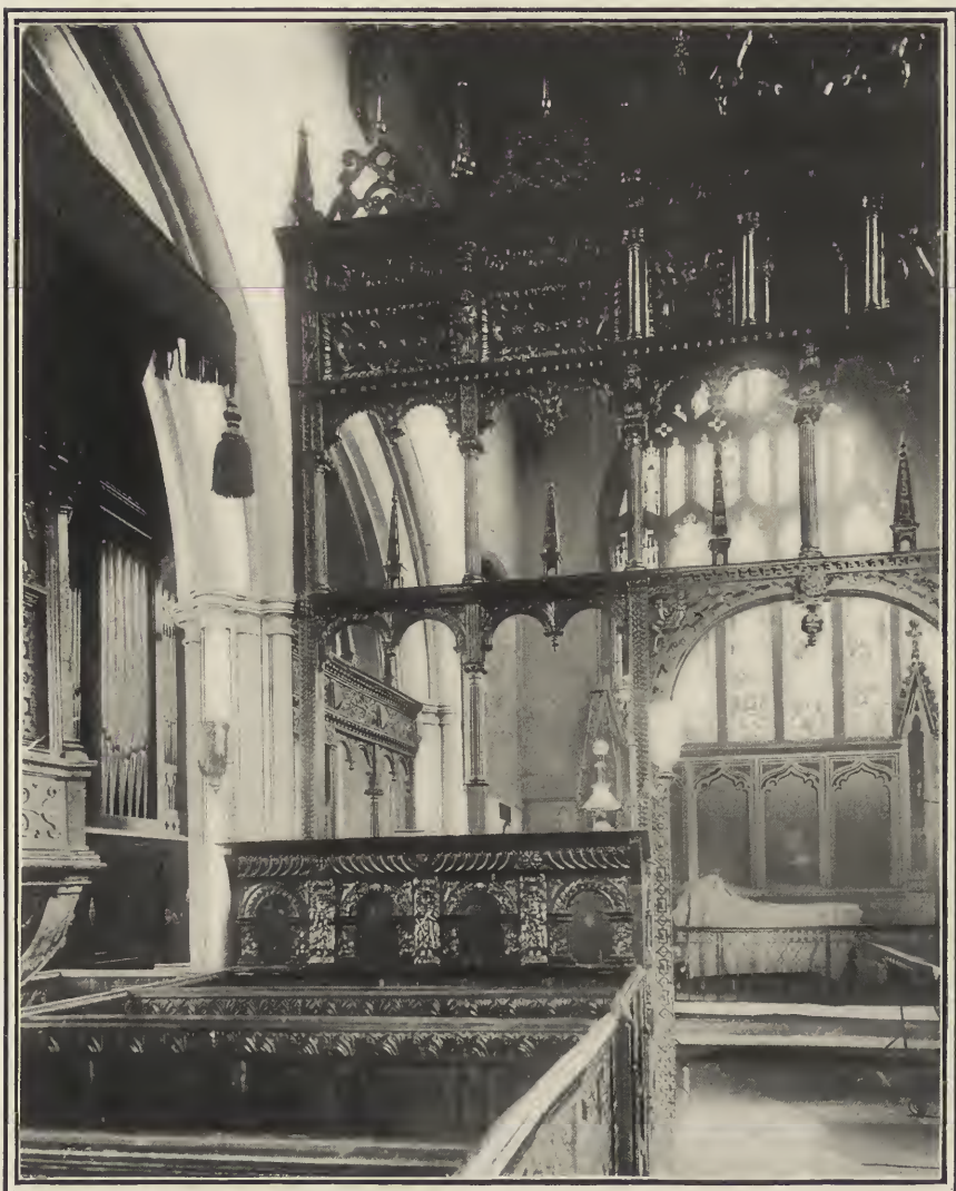
PLATE 5.—Here the northern half of the choir screen can be seen on a large scale, and while the light twinkles and flashes much of the elaborate carvings of the upper members, the work of the enclosure below and of the admirable Jacobean pews next adjoining it can be perfectly appreciated. It is odd to see in so beautiful a chancel, behind one of the most precious choir screens in England, and in front of an east window with intact fourteenth century tracery and glass, some part of which is intact, to see a wretched modern railing of light ironwork without character or significance of any sort in use as the altar rail. That is to say, as the very centre and chief attraction of the whole church to the faithful worshippers and communicants who form part of the congregation.
