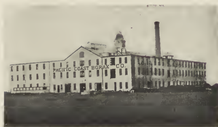
FIG. 5.—FACTORY BUILDING, ERECTED IN 1891.
