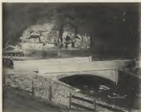
FIG. 8.—BRIDGE ON EVERGREEN ROAD, NEAR PITTSBURGH, PA. Span 28' 0"; Width 20' 0"; Test 12-Ton Roller.
