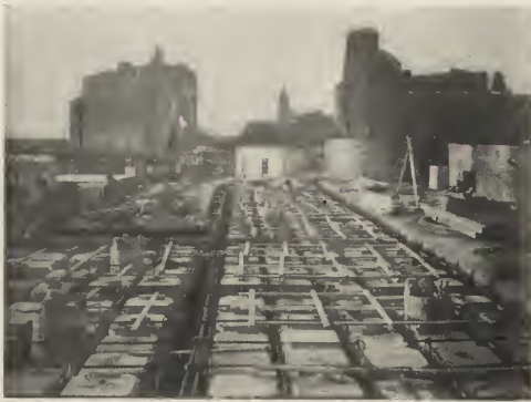
FIG. 31.—THE FLOOR SHOWN IN FIG. 30 IN PROCESS OF CONSTRUCTION.
