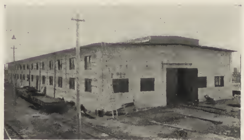
FIG. 34.—CONCRETE WALLS FOR BLACKSMITH SHOP.
