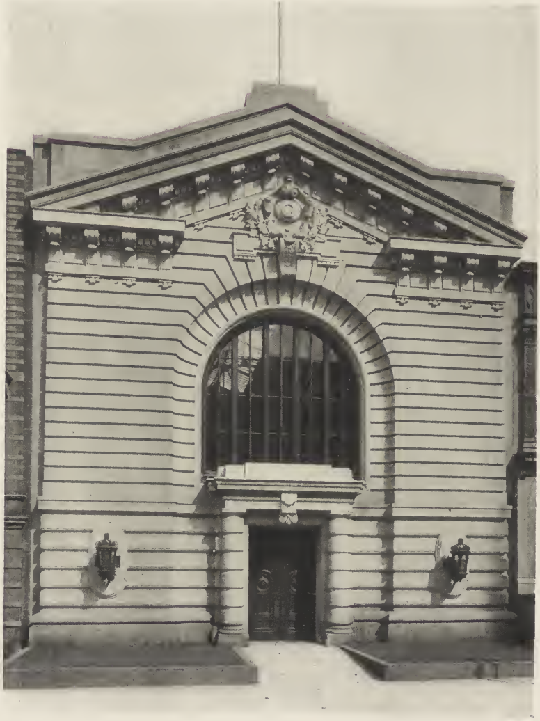
THE RIDING STABLE OF FRANK GOULD. 57th Street, New York City. York & Sawyer, Architects.
