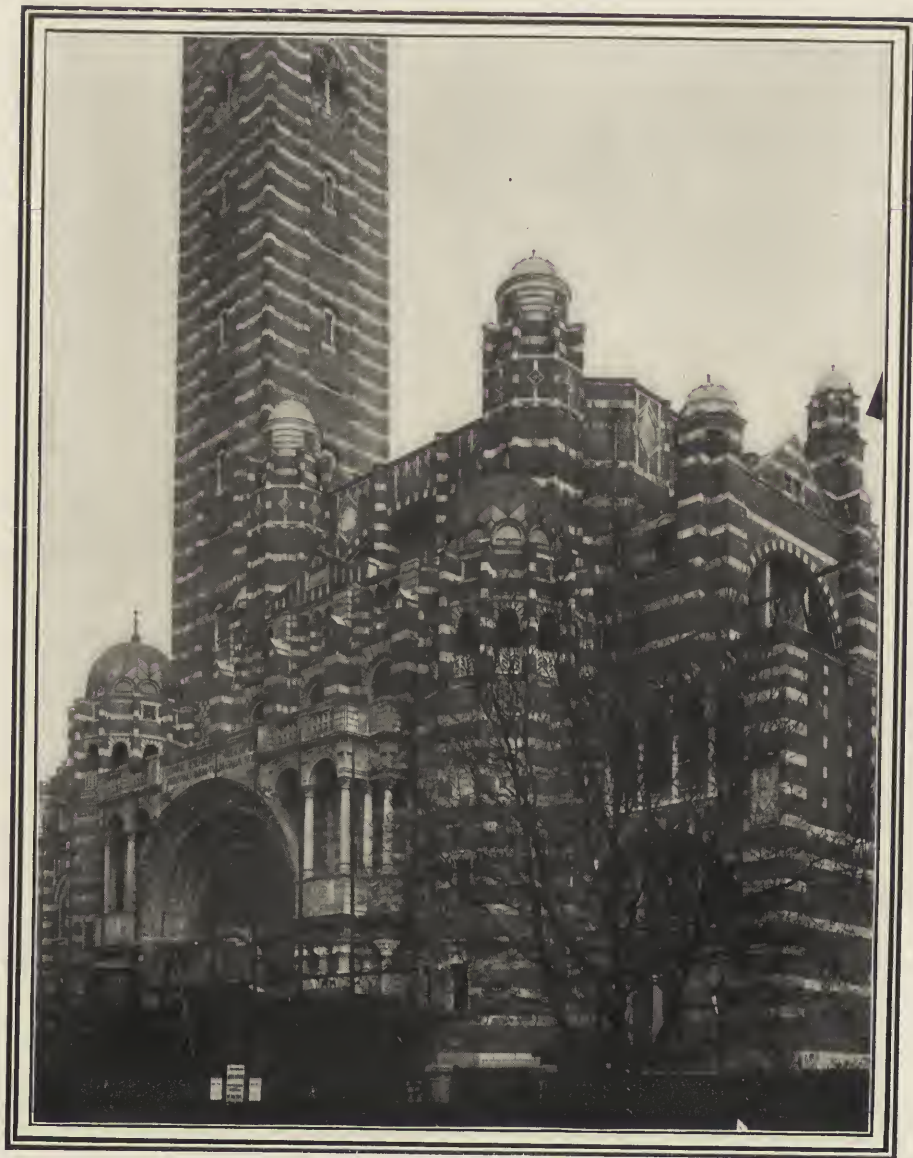
ANOTHER VIEW OF THE WEST FRONT OF THE NEW CATHEDRAL AT WESTMINSTER, SHOWING THE SUCCESSIVE PLANES OF PORCH, NARTHEX AND NAVE CAUSED BY NEIGHBORING RIGHTS OF ANCIENT LIGHT. THE TYMPANUM OF THE ARCH WILL BE FILLED WITH MOSAIC.
