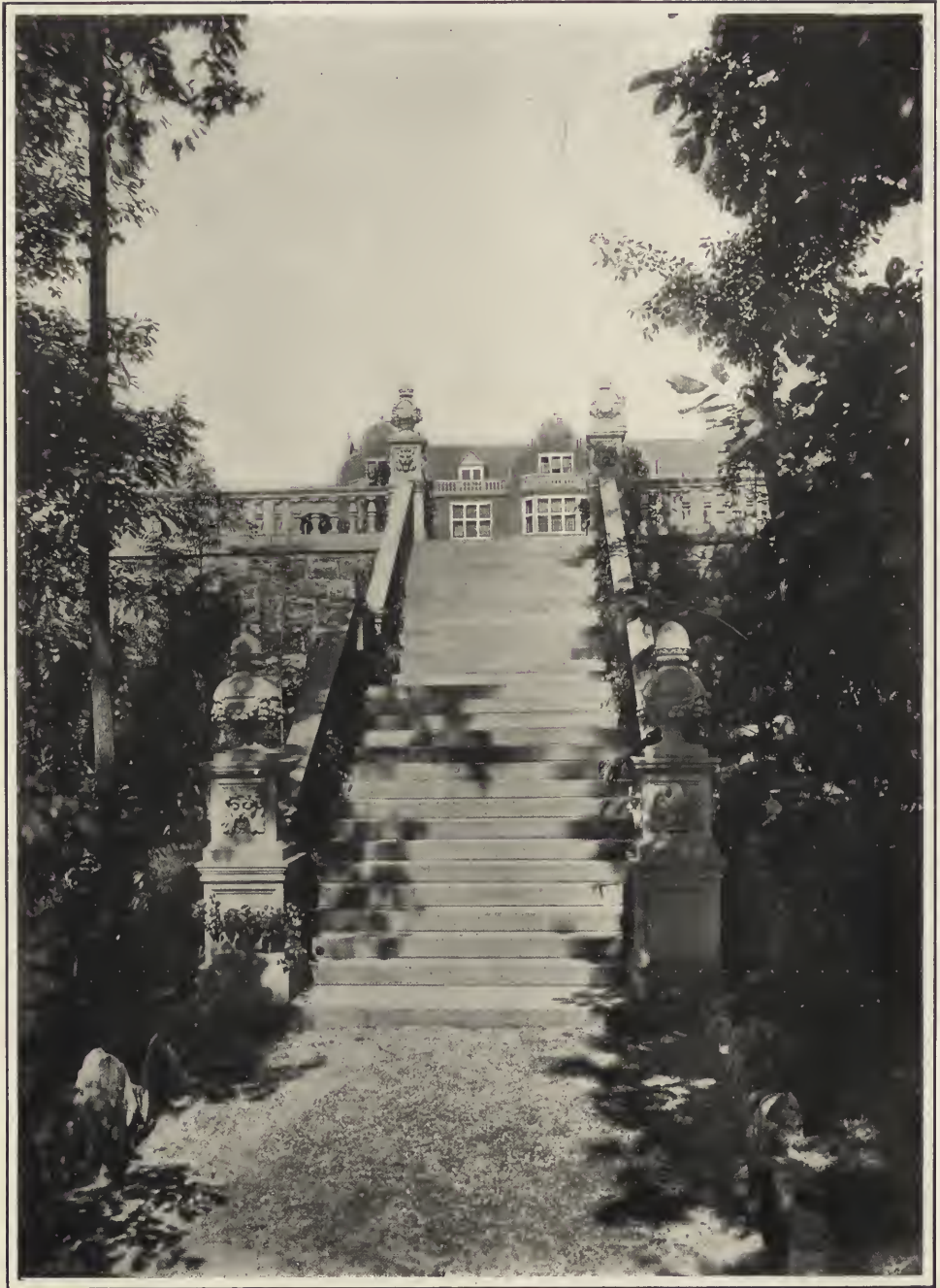
FIG. 5. A STAIRWAY IN THE GARDEN.
