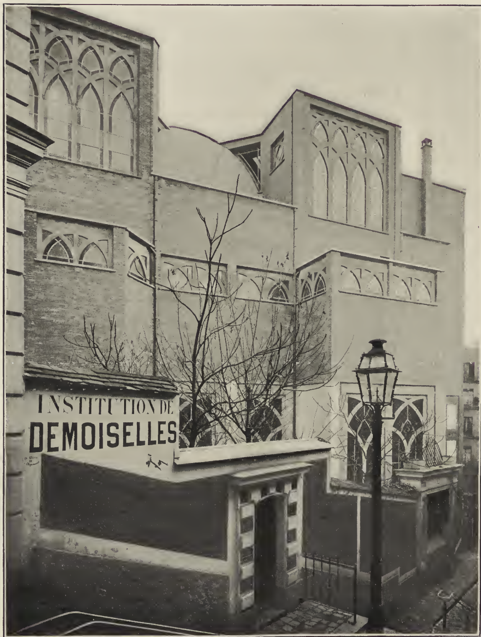
FIG. 4.—ONE OF THE SIDES OF THE CHURCH. Showing the Scheme of Construction Adopted.
