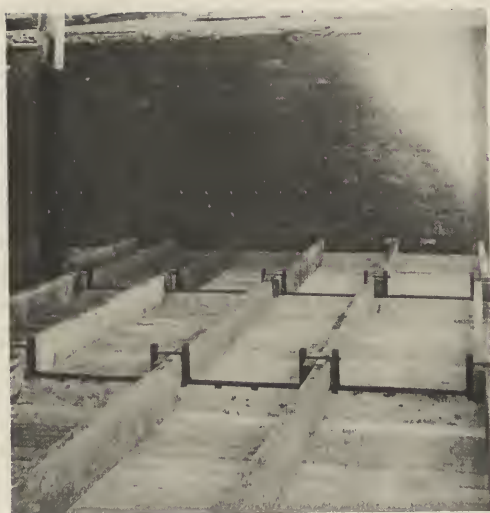
FIG. 27.—CENTERING FOR A STEEL FRAME BUILDING WITH REINFORCED CONCRETE FLOORS.
