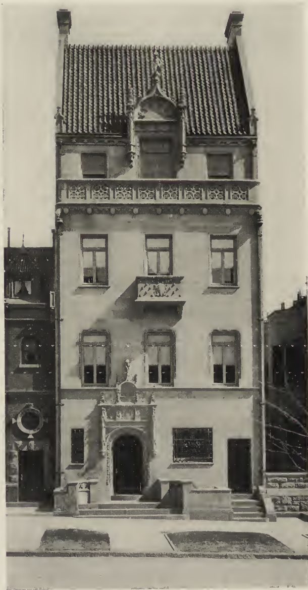
RESIDENCE OF J. N. JAROS, ESQ. No. 266 West End Ave., New York City. R. L. Daus, Architect.
