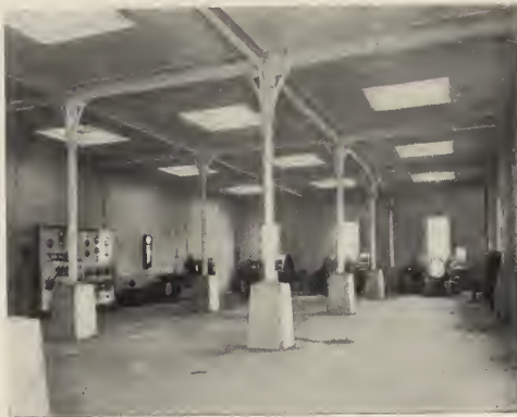
FIG. 38. INTERIOR VIEW OF ENGINE ROOM OF C. R. R. WORKS AT ELIZABETHPORT.
