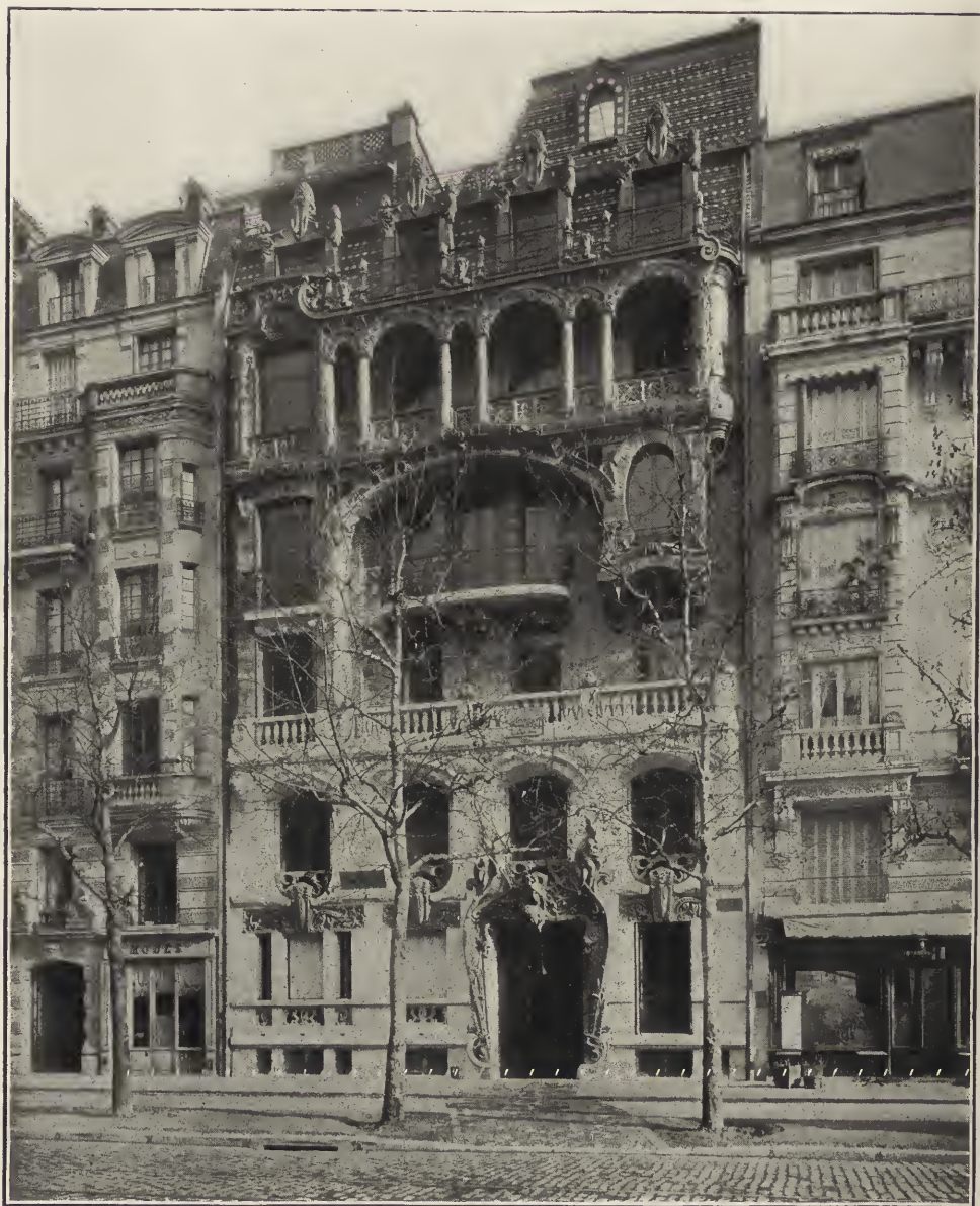
FIG. 1. AN APARTMENT HOUSE IN PARIS DESIGNED BY M. LAVIROTTE AND CONSTRUCTED ABOVE THE SECOND STORY OF BRIQUE ARMÉE.
