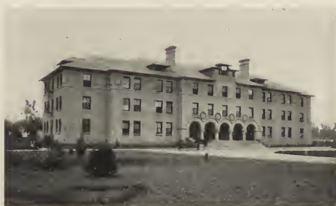
FIG. 7.—GIRLS' DORMITORY AT PALO ALTO, CAL.
