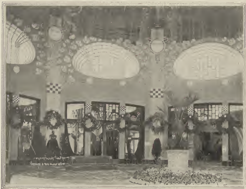
INTERIOR OF THE CENTRAL ROTUNDA.
