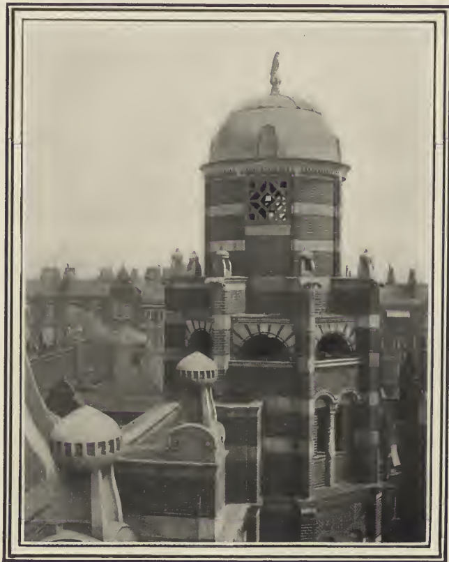
THE UPPER PORTION OF THE STAIR TURRET FLANKING THE APSE.
