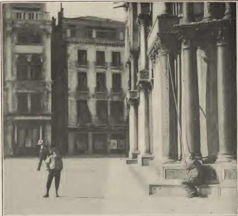
FIG. 12. THE LEANING COLUMNS OF S. MARK'S FAÇADE, VENICE.
