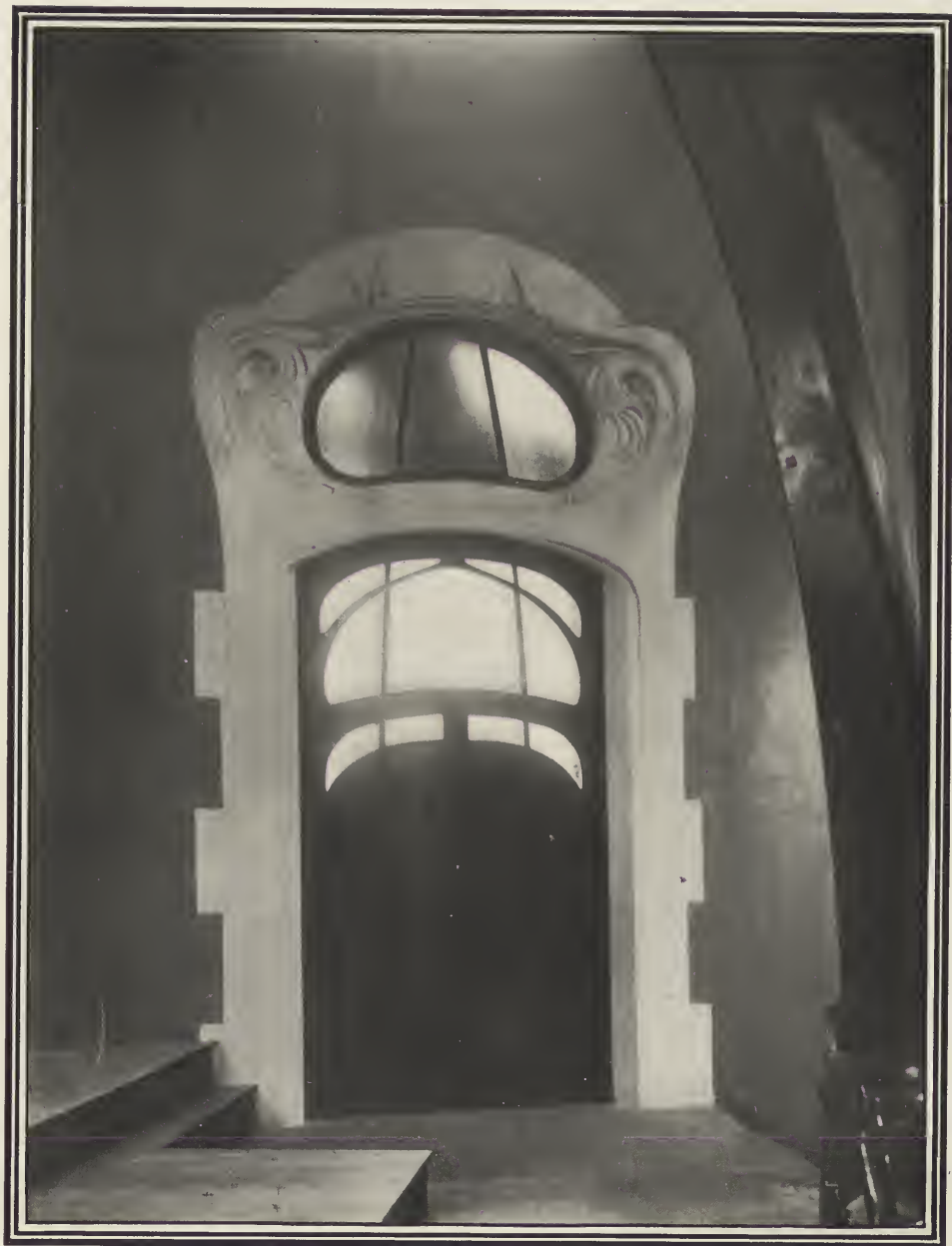
DOORWAY LEADING FROM THE HALL.
