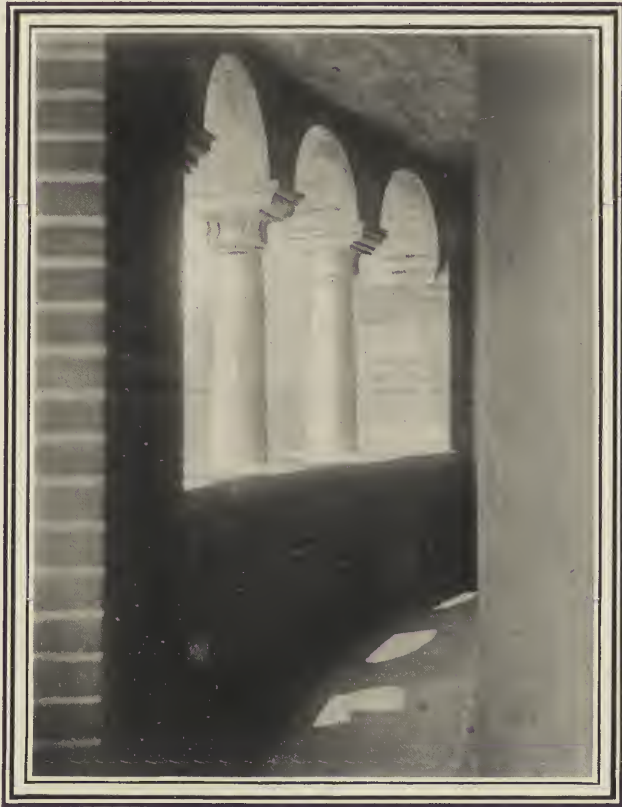
PASSAGE OF THE EXTERNAL GALLERY ABOVE THE VAULT OF THE APSE. THE COLUMNS HAVE THEIR BASES UPON A STRING-COURSE BELOW.
