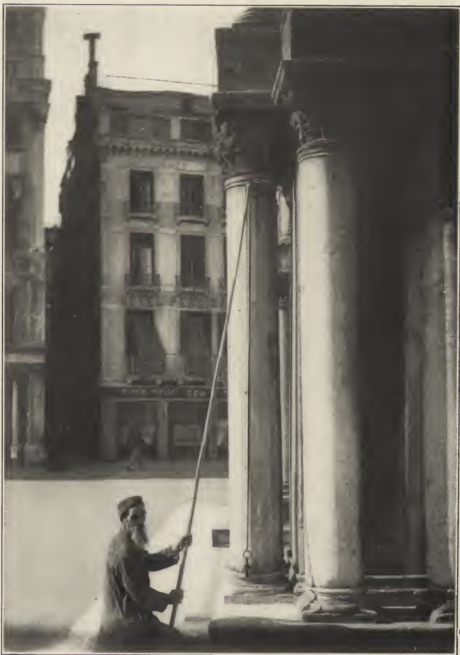
FIG. 13. THE LEANING COLUMNS OF S. MARK'S FAÇADE, VENICE.
