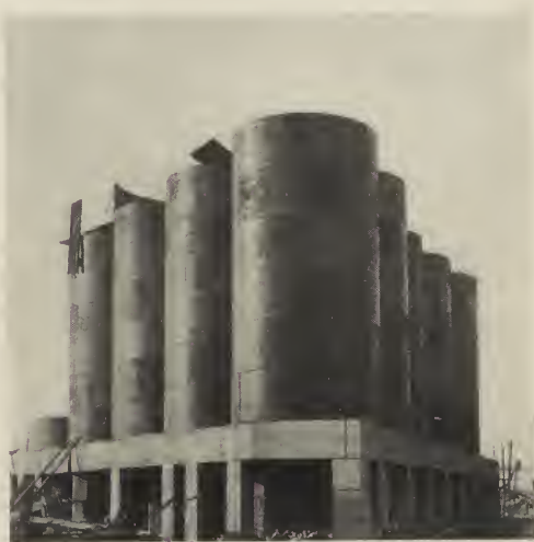
FIG. 30.—FLOOR FOR THE SUPPORT OF GRAIN BINS.
