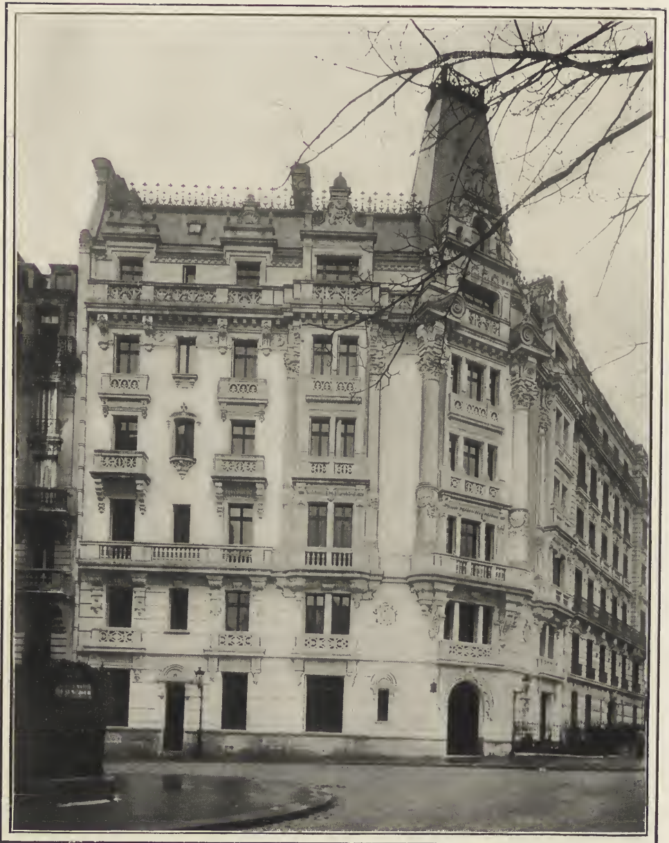
FIG. 11.—APARTMENT HOUSE ON THE BOULEVARD BEAUSEJOUR.
