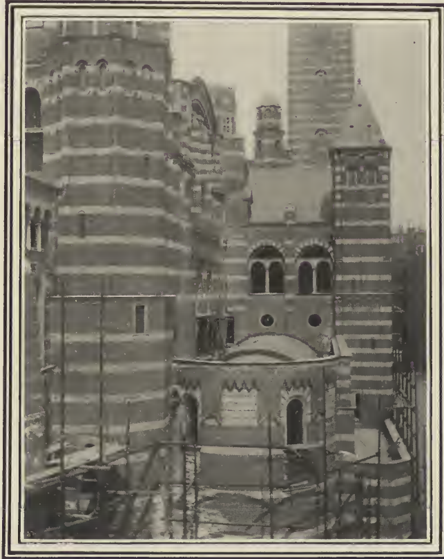
NORTH TRANSEPT OF THE NEW CATHEDRAL AT WESTMINSTER, FROM THE EAST, SHOWING ALSO THE CONCRETE BARREL ROOF TO THE LADY CHAPEL.
