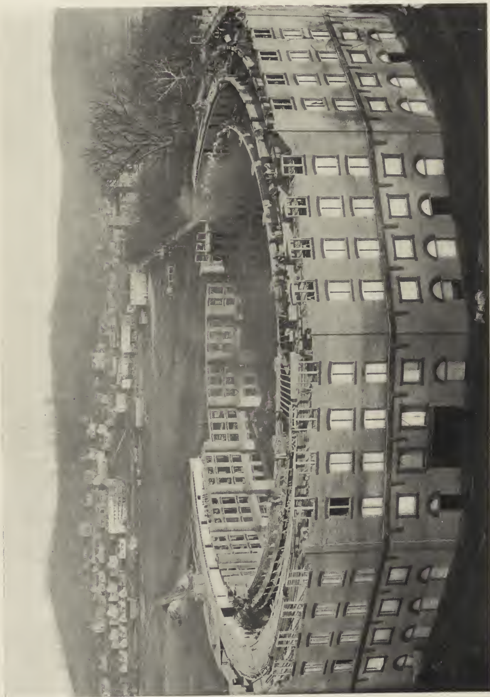
FIG. 24.—A HOTEL AT WEST BADEN, IND. All the floors are reinforced concrete. The walls are of brick.
