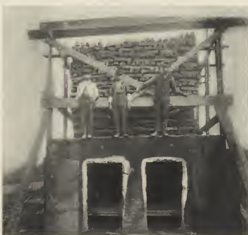
FIG. 22.—FIRE TEST OF CINDER CONCRETE.
