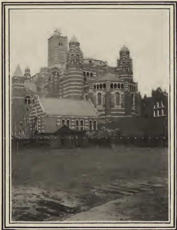
THE NEW CATHEDRAL AT WESTMINSTER, FROM THE SOUTHWEST.
