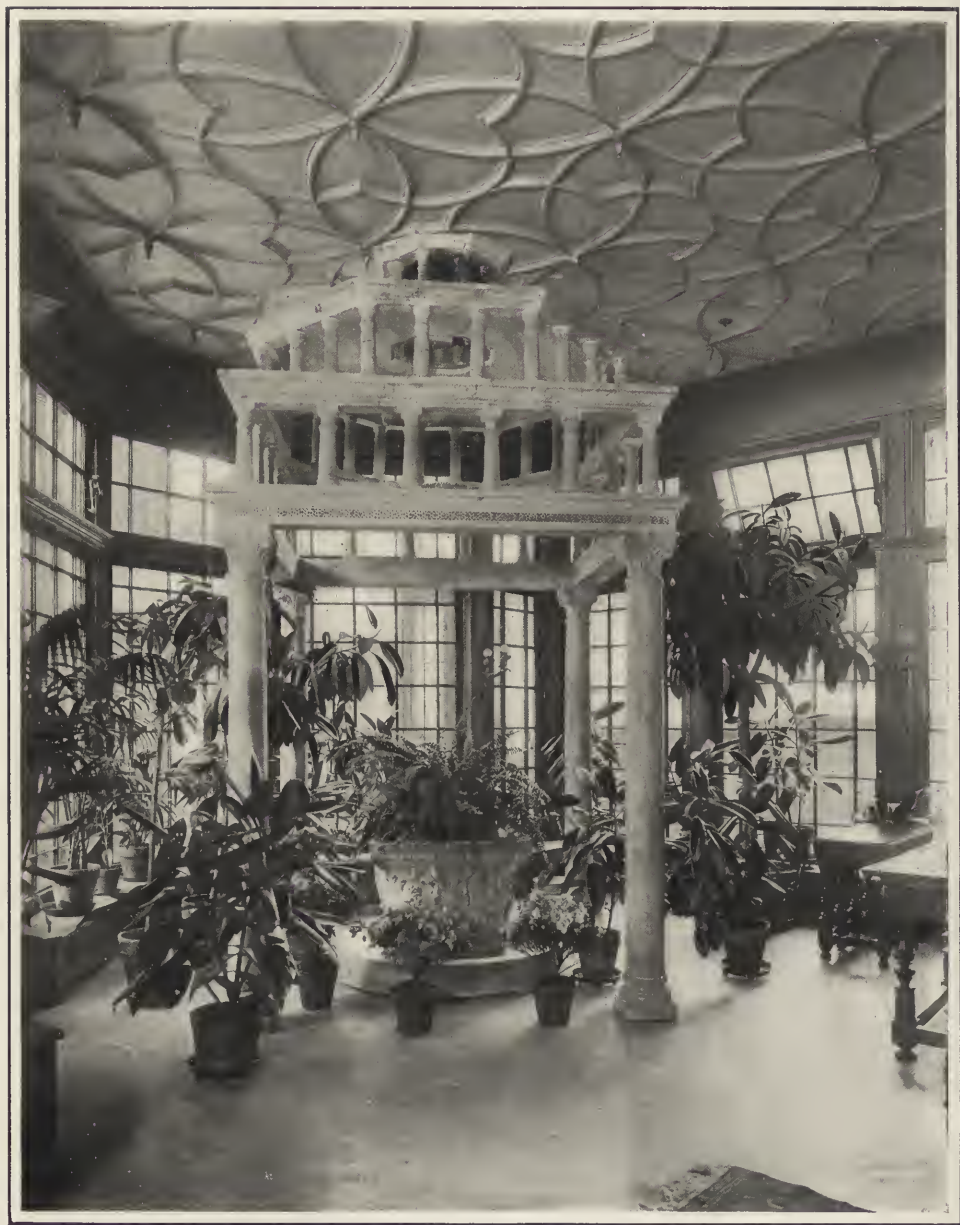
THE CONSERVATORY LEADING OFF THE DINING ROOM.
