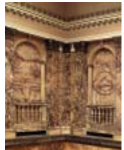
Decorative 'marble' detail in the foyer of Northumberland House
