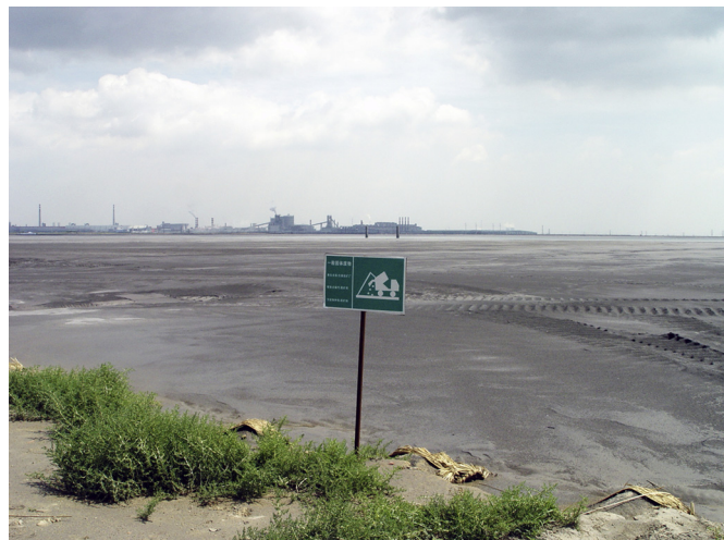
Fig. 3. Photograph of the Baotou tailing dam.
