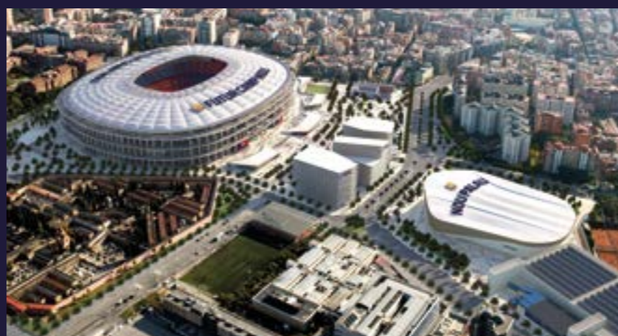
ORIGINAL PLAN Virtual image of the current plan for Espai Barça, detailing Camp Nou, the Palau and the Campus Barça.
