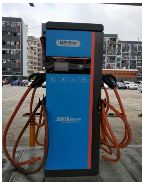
Figure 5 Charging terminal with four chargers
