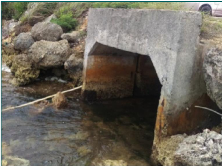
Plate 16: Drainage Outlet, Neiafu, Vava'u
