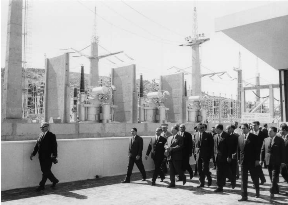
Presidents Tito and Nasser visiting the building site of Aswan Dam, Egypt 1968
