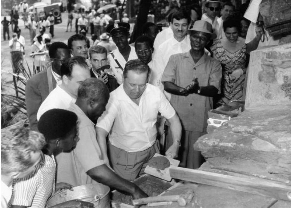
President Tito laying foundation for the new hydroelectric power plant in Kpime, Togo 1961
