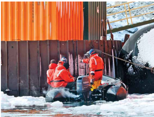
Figure 4.29. The Blue Ribbon Panel inspecting the Palmer Station pier. Source: Craig Dorman.
