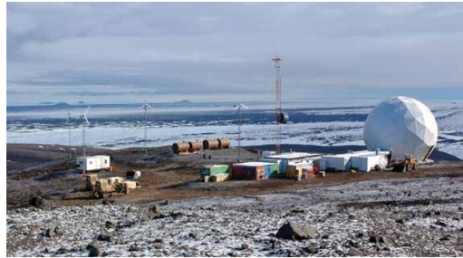
Figure 4.61. Black Island Telecommunications Facility. Source: Steve Martaindale.
