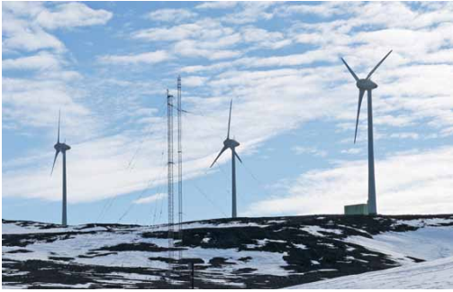
Figure 4.52. Wind turbines at McMurdo Station. Source: Craig Dorman.
