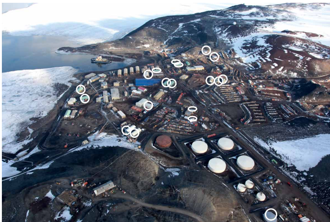
Figure 4.47. Photo of McMurdo Station showing the diversity and geographic spread of USAP warehouses (circles). Source: George Blaisdell.
