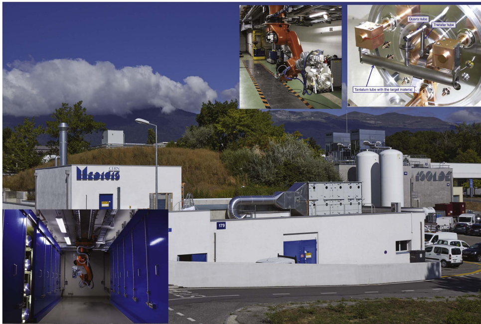
Figure 3. The ISOLDE ‘hot’ area with the new MEDICIS building. The upper insets are (left) the robot used for target manipulations and (right) an ISOLDE target without vacuum container. The inset in the lower part of the figure shows the target storage shelves in MEDICIS.
