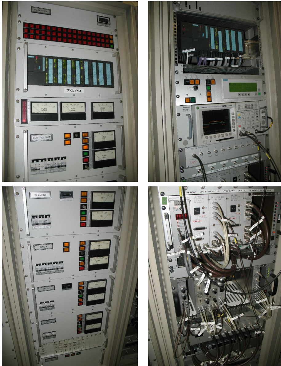
Figure 22: REX amplifier for the 3 rd 7-gap resonator, showing the two racks (each cut in two by the photograph).
