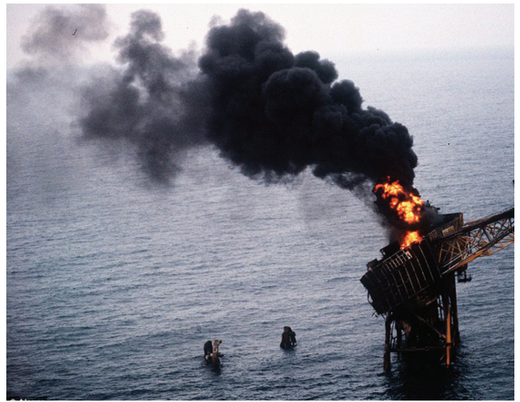
Figure 3. The remaining oil wells module continued to burn for weeks until famed firefighter, Red Adair, and his team extinguished the remains. Source: BBC.
