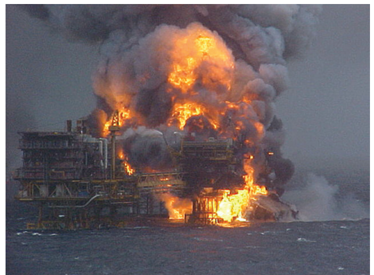
Figure 2. The smoke reached hundreds of feet above Piper Alpha, preventing rescue helicopters from approaching. Source: Technologism.net.
